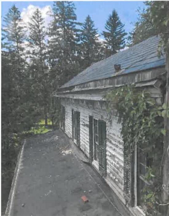
Servant's Wing Porch Roof and Gutter
