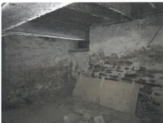
Ductwork to be Removed
