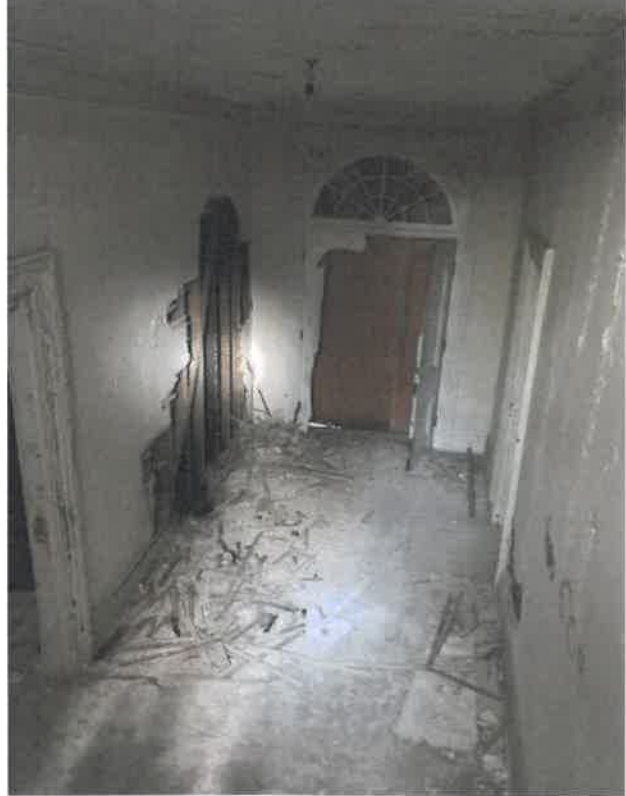
Main Stair Hall
