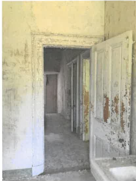
Front Bathroom through Main Stair Hall
