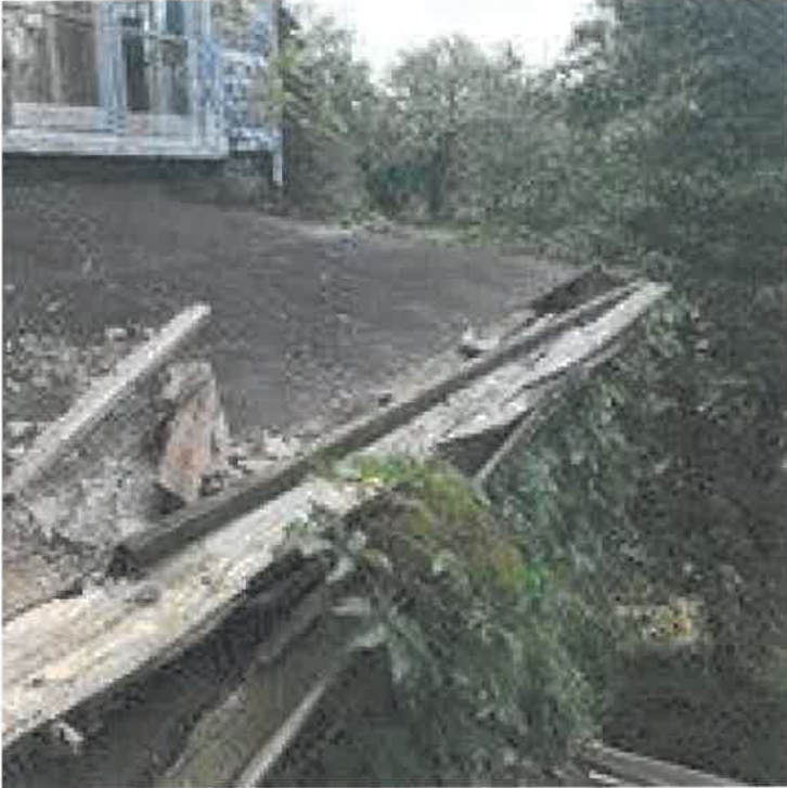
West Porch Roof at Rear of Sun Room
