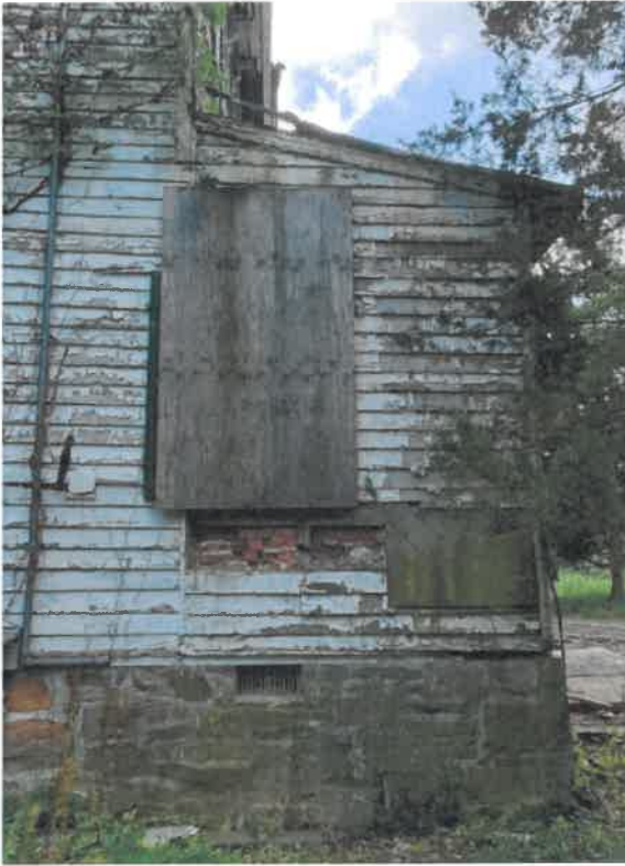
Servant's Wing North West Corner
