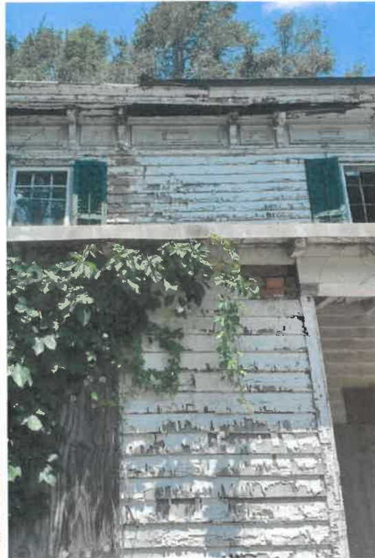
Servant's Wing West Side Soffit and Fascia
