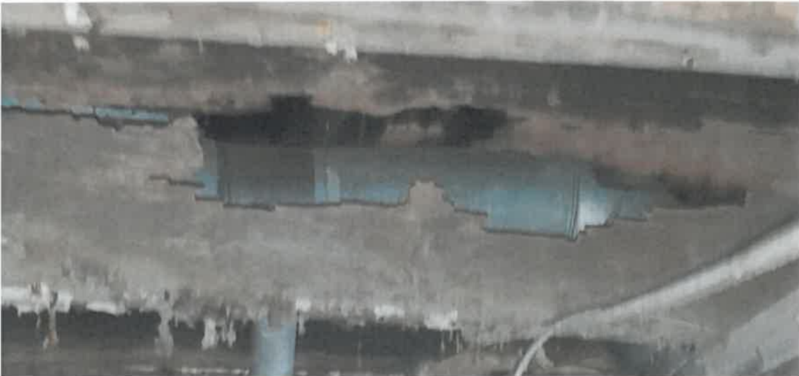
Floor Joist under Dining Room
