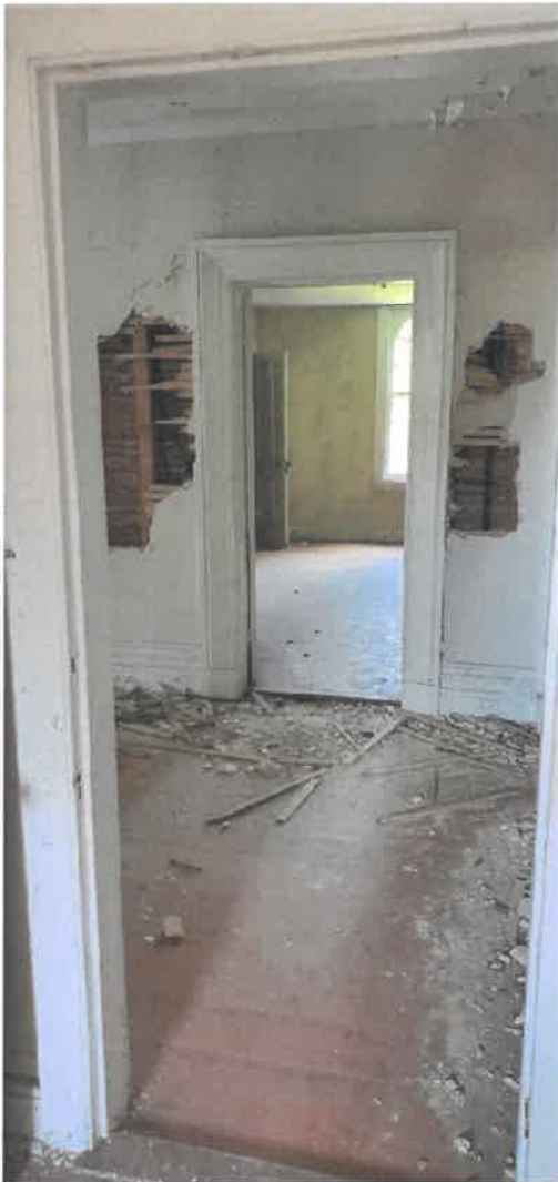
View from East Room to West Room
