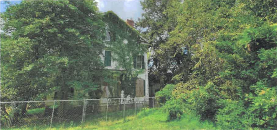
East Side of House
