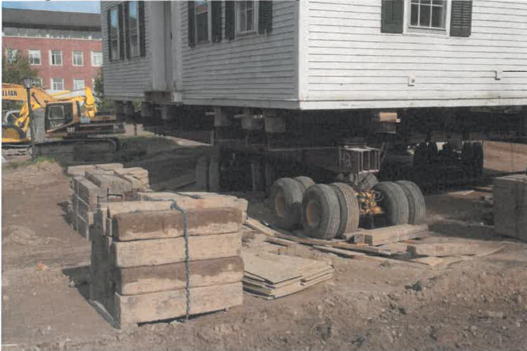
Cribbing stacks in foreground and dollies with steel beam atop
