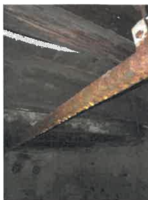
Steel Pipe to be Removed
