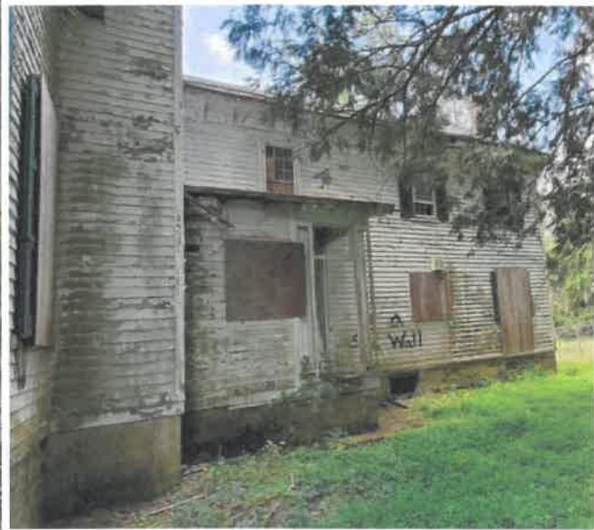
Servant's Wing Showing East Porch and Elevator
