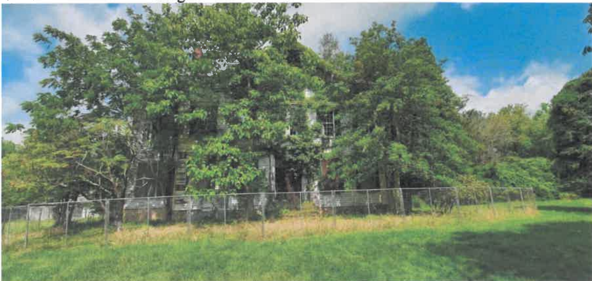
View of Front of the House Showing Overgrown Shrubbbery
